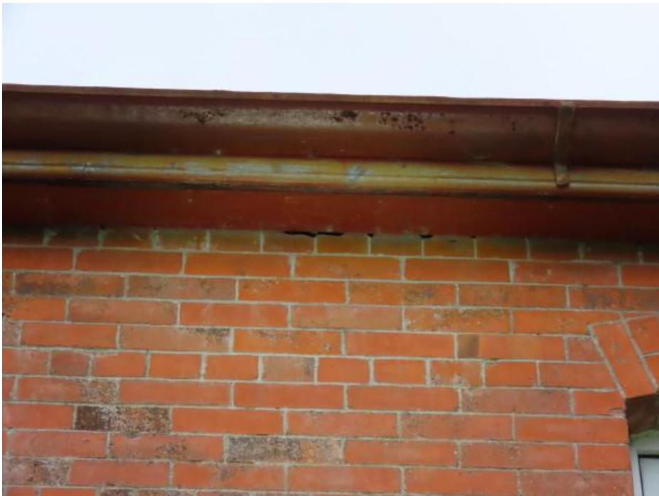
Photo 4 – example of gap at top of walls between bricks and fascia where bats could gain entry
