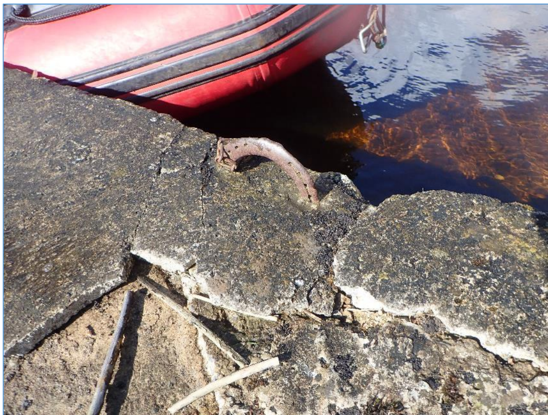
Plate 14: Detail showing horseshoe re-used as pier furniture for tying-off vessels.
