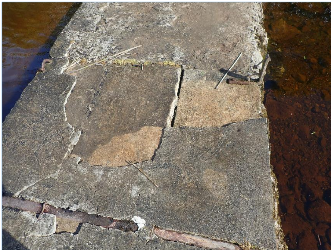
Plate 13: View looking at the join between the older part (top) of the northwest pier and the later addition (centre and bottom).
