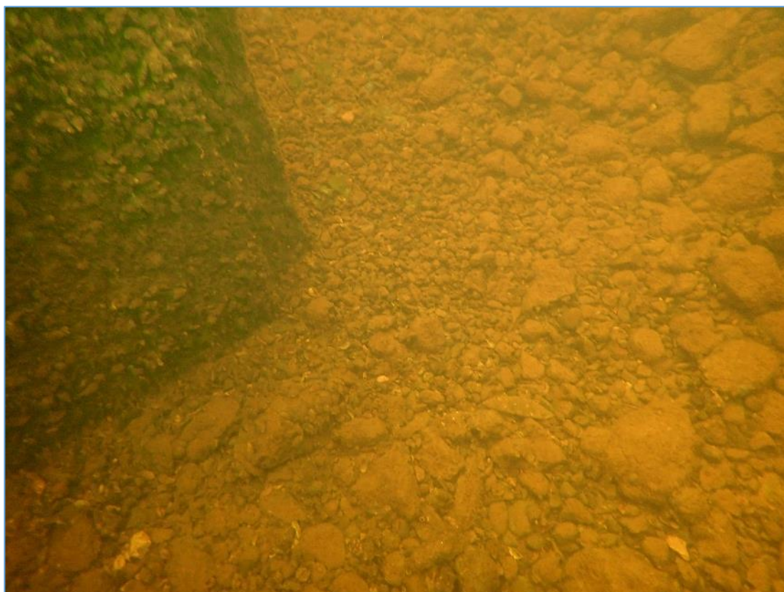
Plate 20: Underwater view showing interface between the base of the northwest pier and the lakebed.
