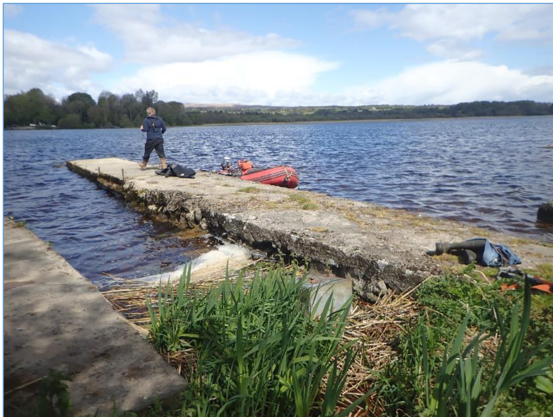
Plate 11: View looking at the northwest pier from the south. The earlier construction phase is clearly distinct from the later component added to the lake side.
